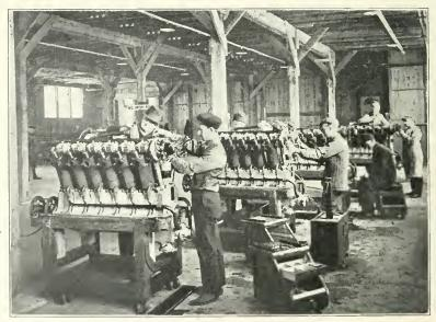
Photo from Packard Motor Car Company ADJUSTING IGNITION SYSTEM OF LIBERTY ENGINES
