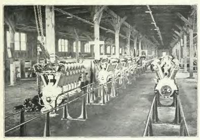
Photo from Packard Motor Car Company LIBERTY ENGINES READY FOR SHIPMENT
