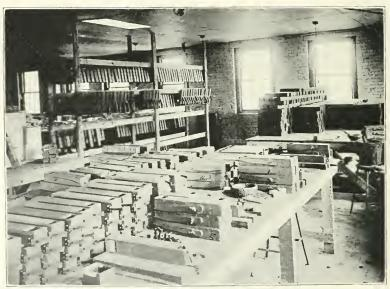
Photo from Penn Toy Company MANUFACTURING TRENCH PERISCOPES
